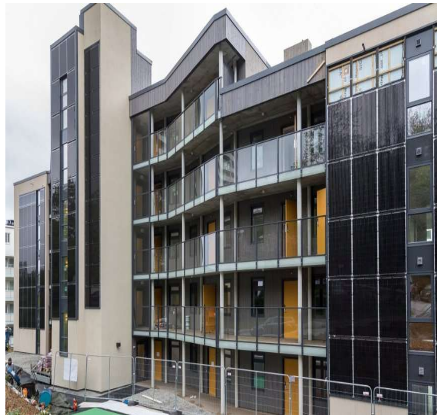
First apartment building BIPV, 42 kW, Norway
