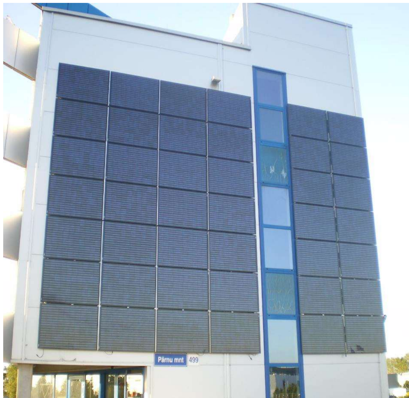
Baltic Disk integrated facade, 12 kW, Estonia
