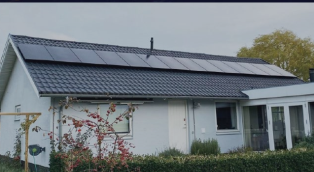
Residential Off-grid ESS
