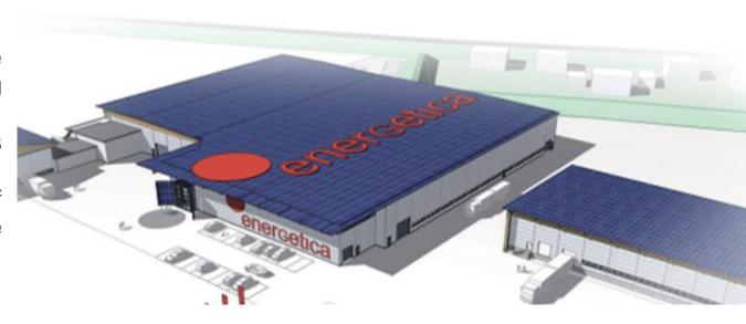
The production process is completely **CO2 emission FREE**. The facility is powered by a 2.6 MW PV plant built with our own smart modules, the adjacent hydro power plant and from adjacent Biomass Energie Kärnten for wood-fueled heating.
