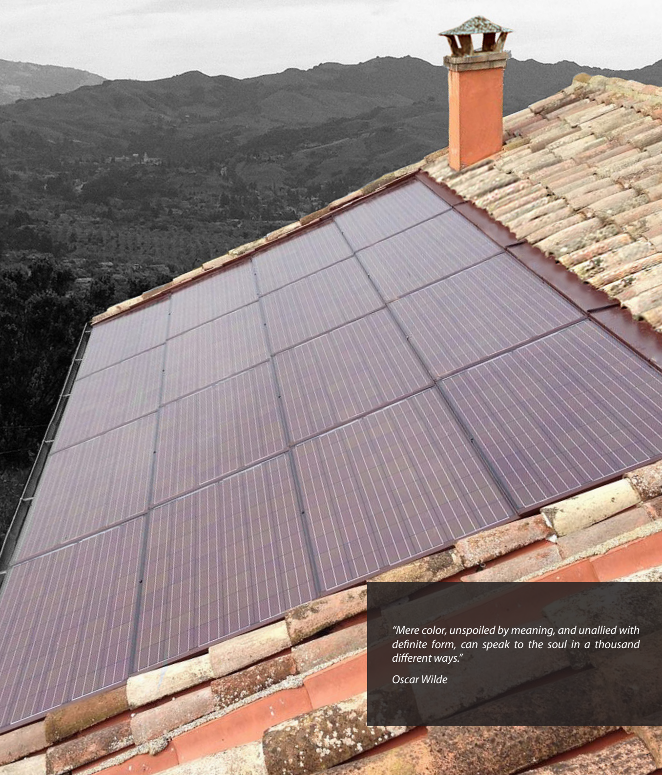
Detail of special BIPV (Solrif®) frame
