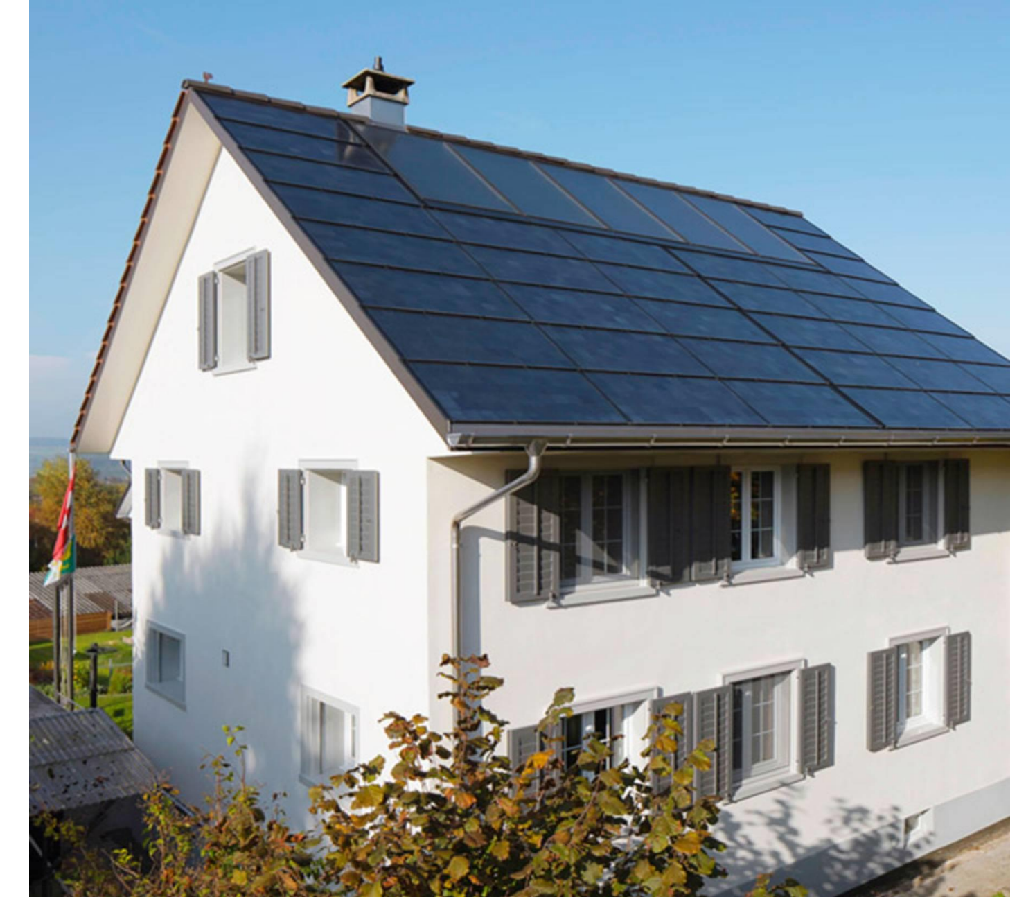
Solrif® system, 10 kW, Switzerland
