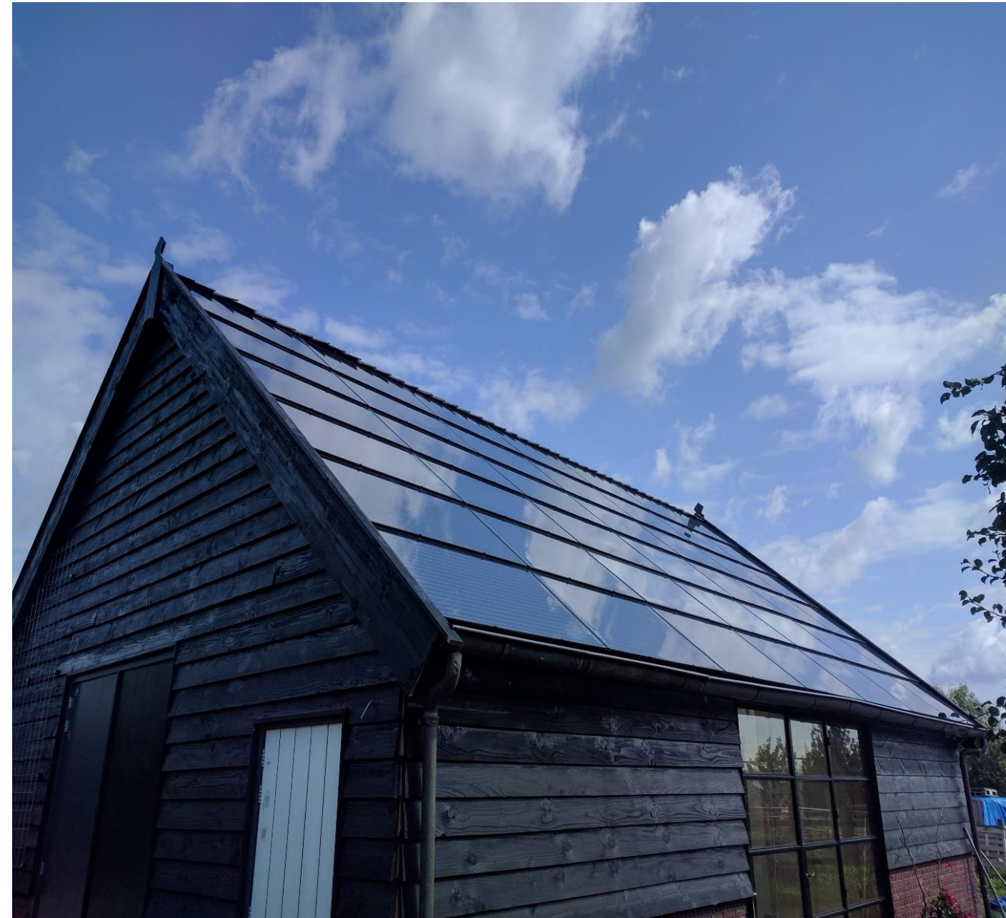
Solrif® system, 10 kW, Netherlands
